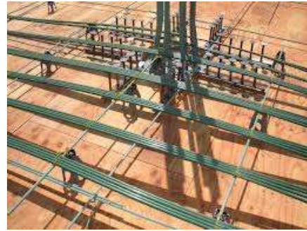
• Mono strand post tensioning reinforcement
